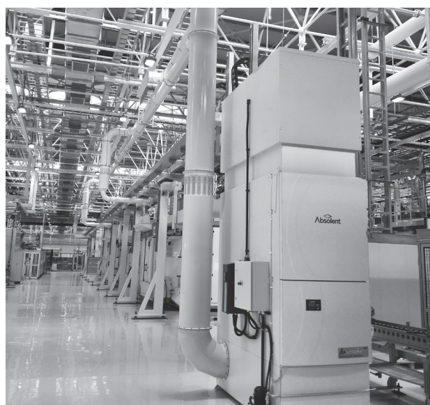
Absolent installation at Volvo Zhangjiakou. Solution: A•smoke80TF (one filter unit for several machines)
